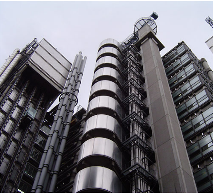
View of Lloyd's building showing exterior vertical circulation cores. 25
